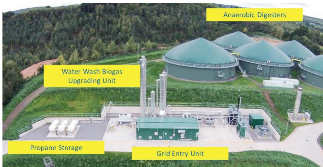
**Figure 9. Biogas plant with biomethane upgrading and gas grid entry point. Also shown is the propane storage required to adjust gas calorific value. Credit: John Baldwin, CNG Services Ltd, UK.**
