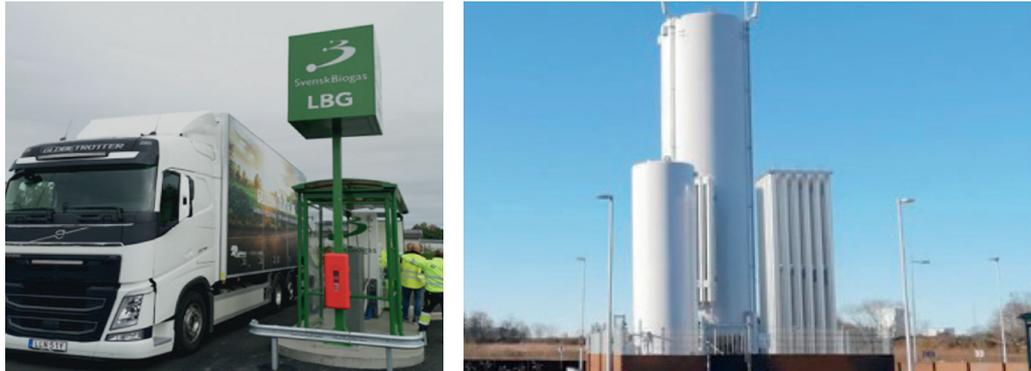
Figure 13. A filling station supplying liquid biomethane. A truck is fueling liquid biomethane to the left, while the picture to the right shows the storage of the liquid biomethane with a cryogenic tank and a vaporizer for the part of the biomethane which is filled as compressed biomethane.
