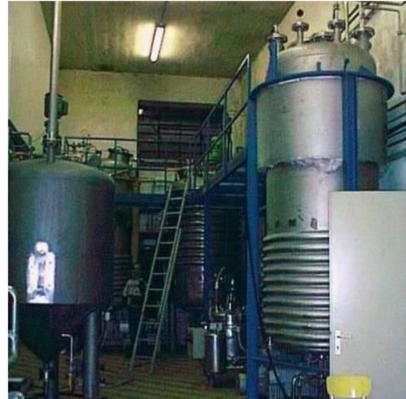
Fig. Biobutanol Testing in an agricultural Bioethanol Facility
